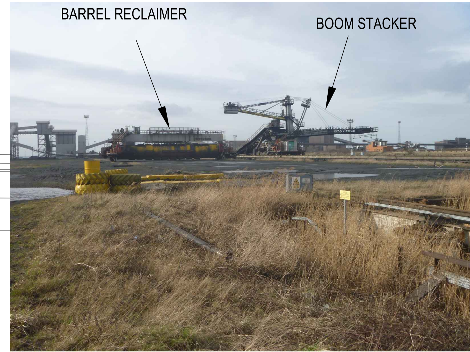
BARREL RECLAIMER AND BOOM STACKER ON SITE TO REMAIN UNTOUCHED
