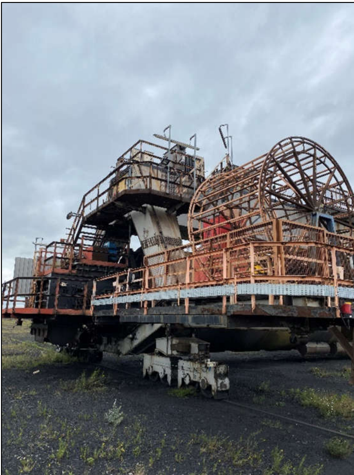
Photograph 4 - Area 10 Reclaimer Stacker
